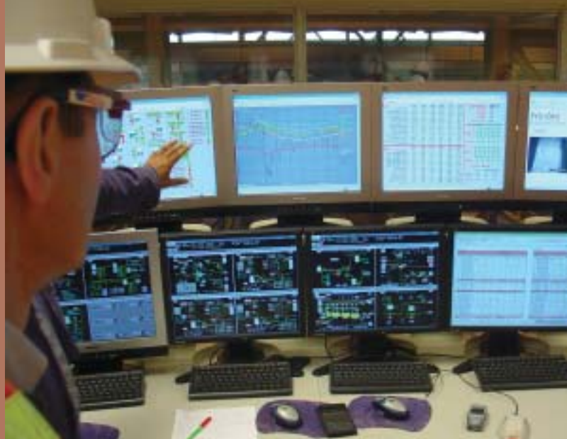
Control room at Antamina concentrator, Peru.
